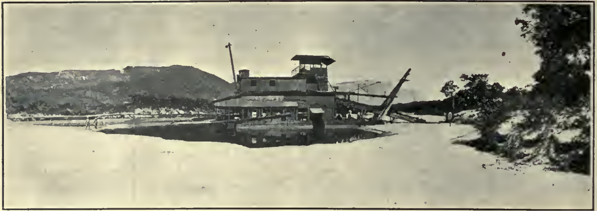
DREDGE IN OPERATION AT MENDANHA.
